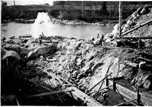
FIG. 4.—EXCAVATING THE TAIL-RACE.
